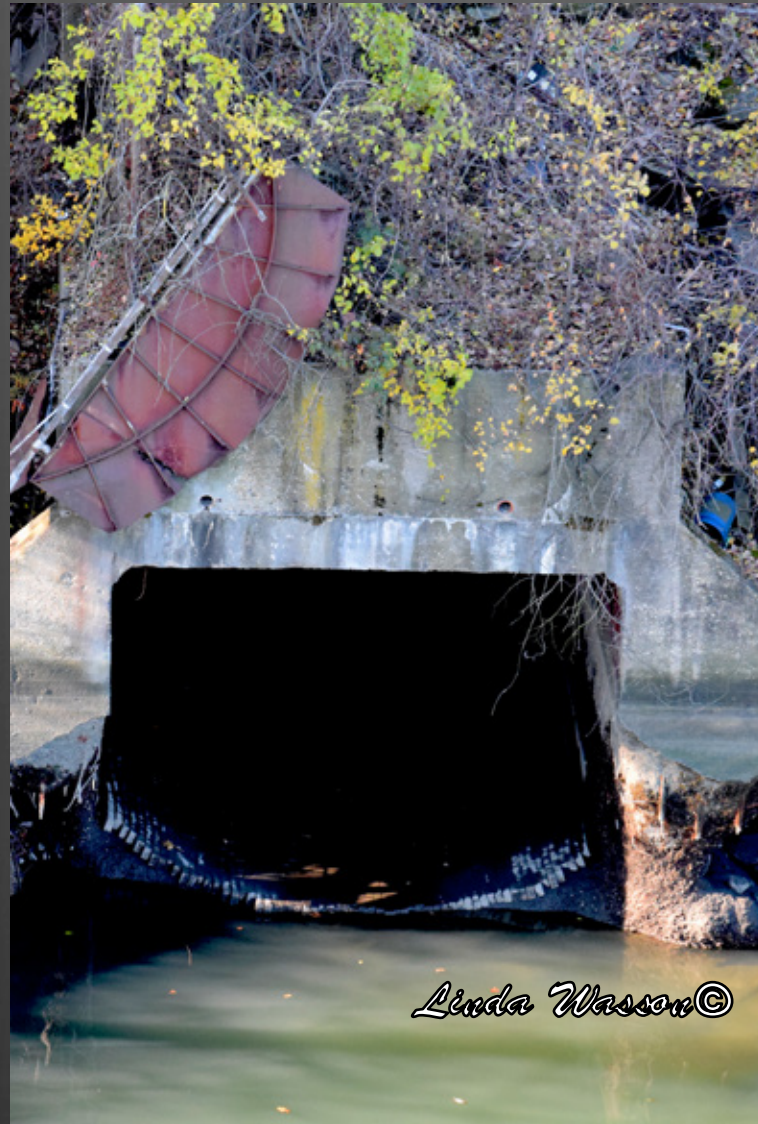
Close up of the Culvert - NE Bank Towards the NW Bank
